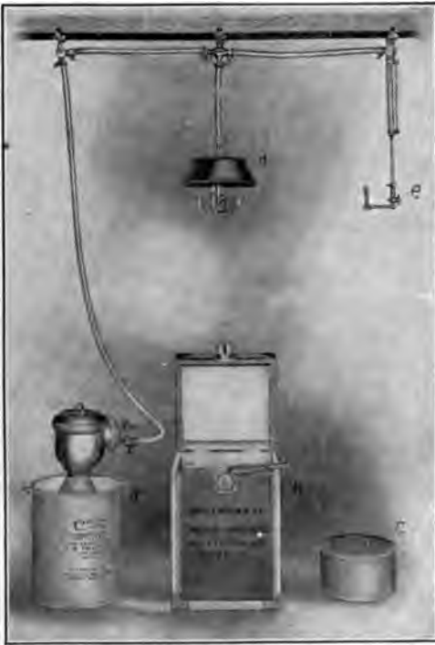
FIG. 160.—Acetylene outfit for field hospital. ( Colt system. )
